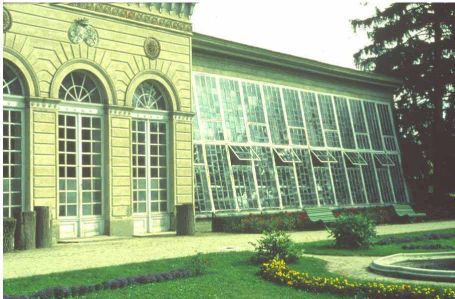
Greenhouse Telc, Czech republic
